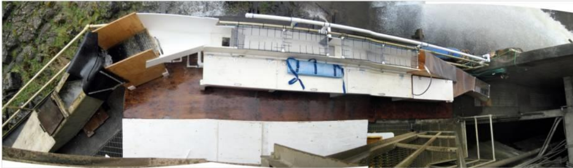
Figure 1. Overhead view of the Denil (left), trap, and ladder return (right) used to collect adult salmon and steelhead at Willamette Falls Dam in 2011-2014.
